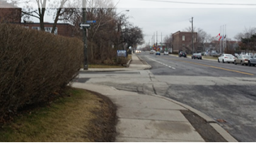
No stop line at Fourth Street and Birmingham Street
