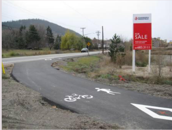
The new multi-use path includes a distinct separation from the road at many points along its length
