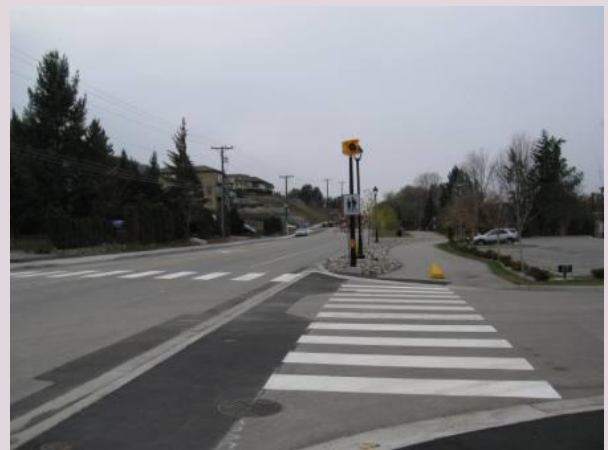
Upgrades included the installation of a multi-use path, crosswalk improvements and pedestrian-activated lights
